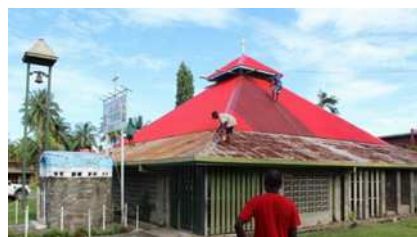
Renovation of the roof of St. Stephan's church at 3 Mile, Lae
