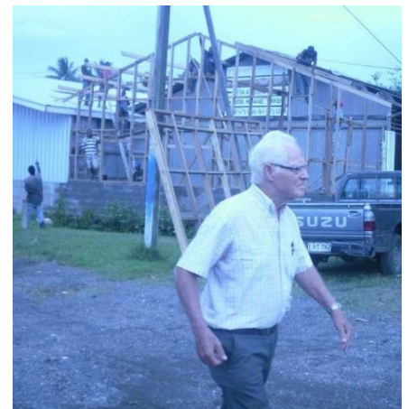
Fr. Sido with at the background extension works at St. Joseph's
