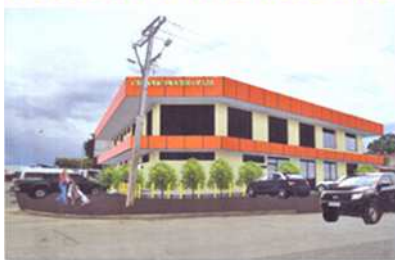
Proposed two-storey Chancery for the Diocese of Lae along the 2 nd street on the ground of St. Mary's Cathedral
